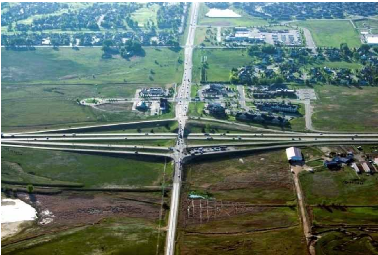
Future improvements to the Interstate 25 and Highway 392 interchange are a result of regional cooperation between the City of Fort Collins, Town of Windsor, and Colorado Department of Transportation.
